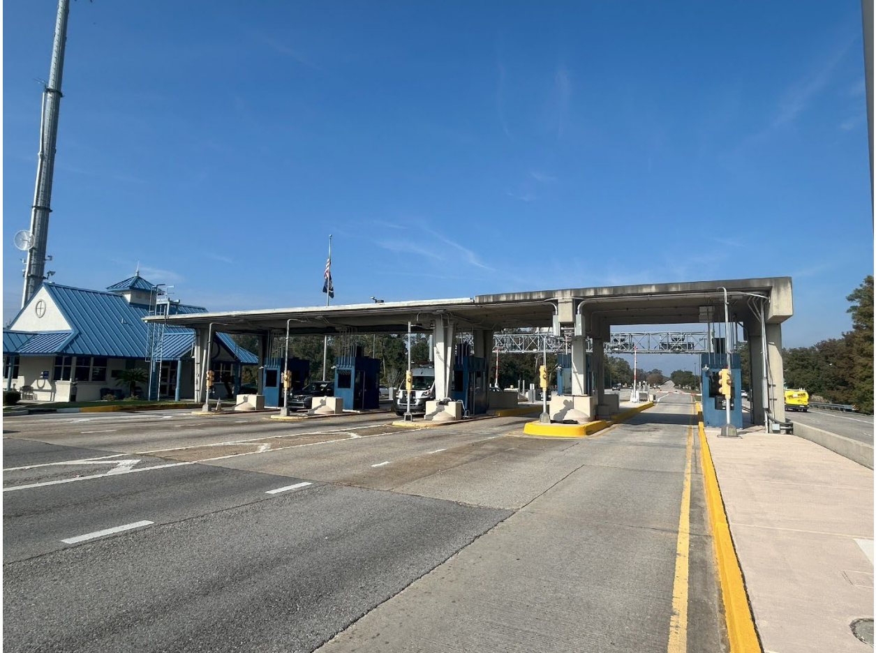
Figure 3 Exit from Toll Plaza
